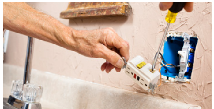
AFCI/GFCI outlets are harder to install than standard outlets. Eliminate them by using Dual Function Circuit Breakers.
